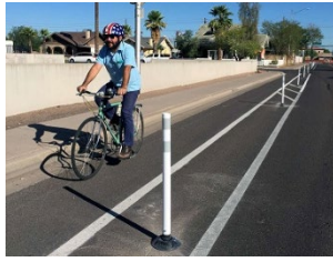
Dedicated Lane with Physical Barrier
